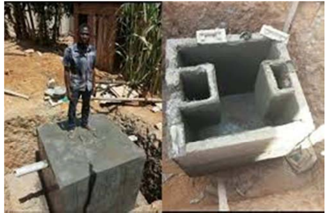
Figure 3. Construction of the biodigester (septic tank) system.
