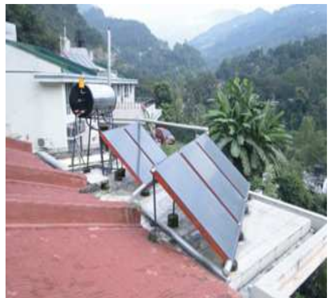
Figure 2. Closed view of thermosyphon type solar water heating system
