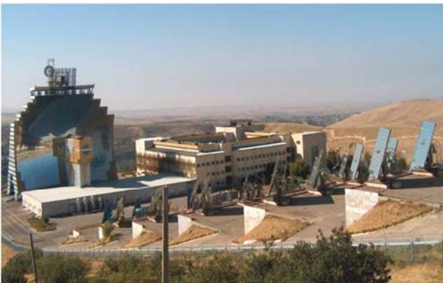
Figure 1. The large solar oven in Uzbekistan with a thermal power of 1000 kW.
