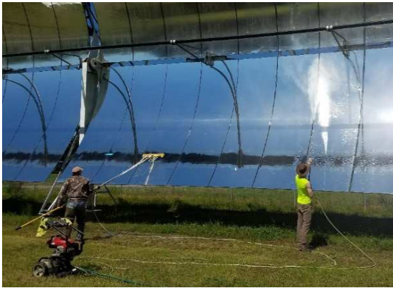
Figure 3. Reflector Washing.
